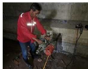
Core Drilling
